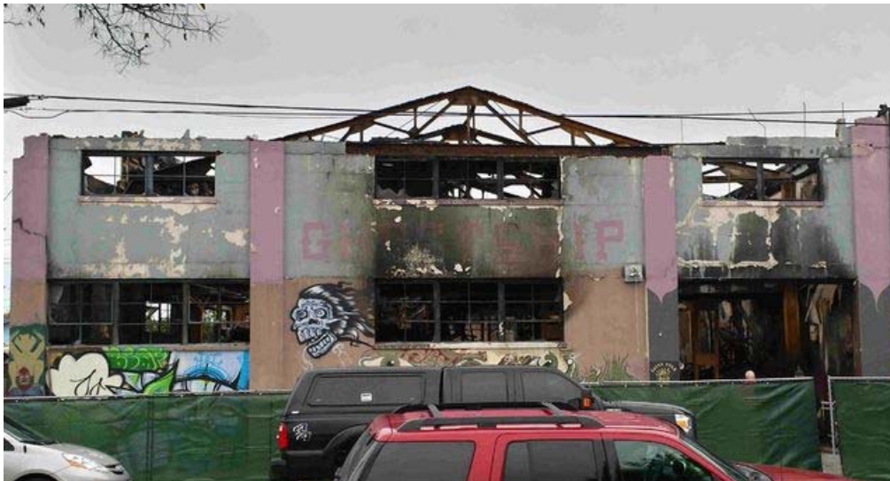
The “Ghost Ship” warehouse that burned down December 2
